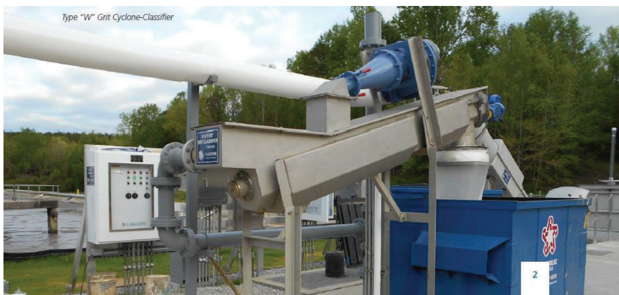
Figure 6 - Lakeside Type "W" Grit Cyclone Classifier
